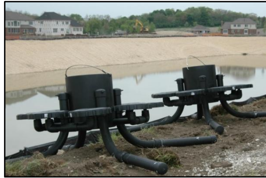
Two MARS Aerators awaiting installation
