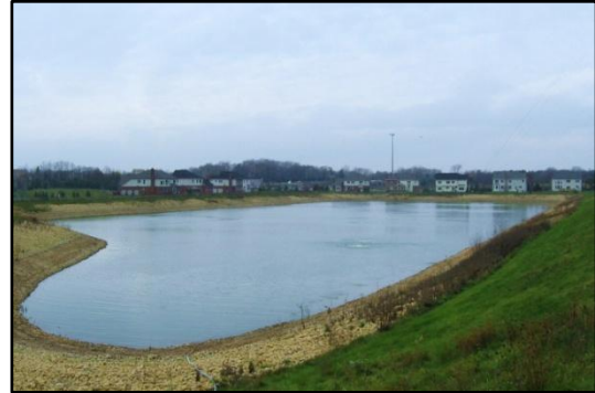
Hawthorne Woods effluent storage lagoon
