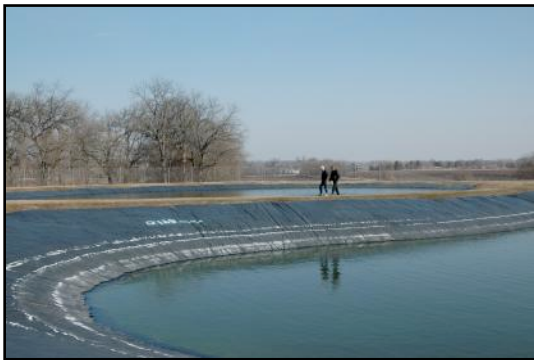
Glenwood Wastewater Lagoons
